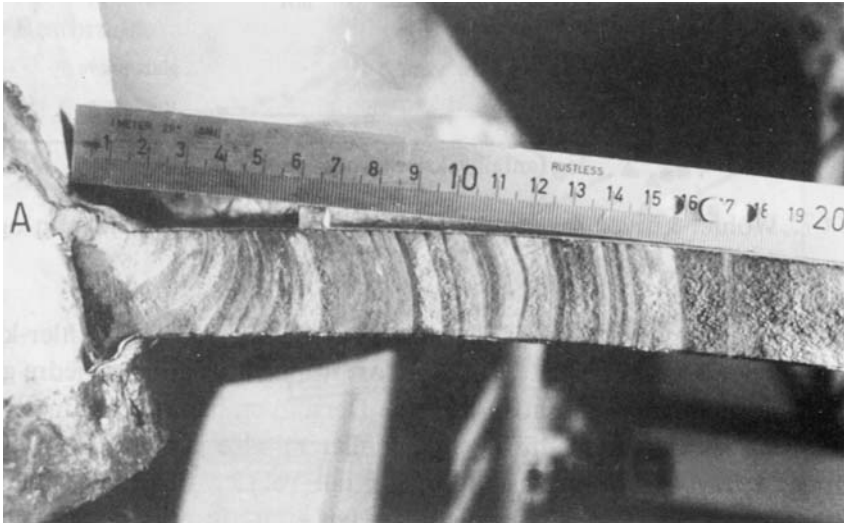
Figure 7.66 Crack surface after fatigue of steel in seawater under cathodic protection. (From the hotel platform “Alexander Kielland”. Photo: B. Lian, Statoil.)
